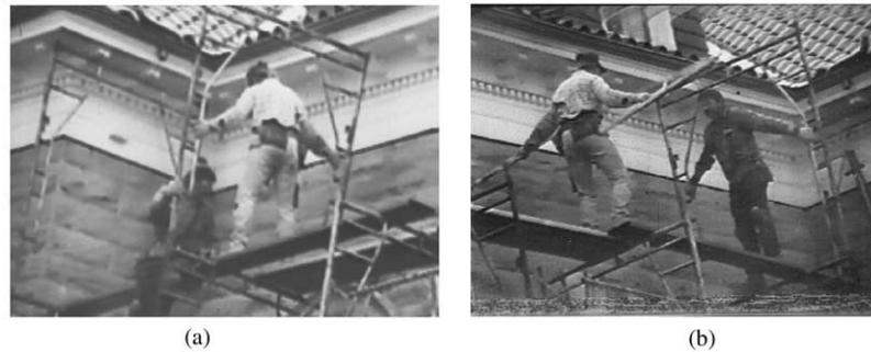
Fig. 1. A great muscle strength can be generated when scaffold workers placed their hands at knuckle height (a). However, once an end frame is lifted out of the lower frame using the method, a fractional force at the anterior–posterior direction plus the weight and the momentum of the top portion of the end frame will pull the workers forward or backward, causing them to become unbalanced and thus increasing their risk of a fall (b).
